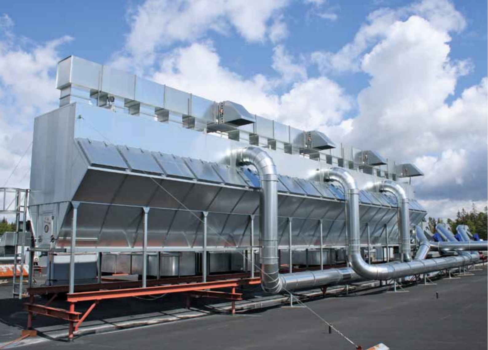
NFKZ3000 Filter with UP venting
