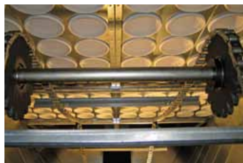
View from the inside of the hopper
