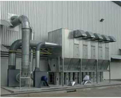
NFP Filter with end inlet and bins for collection
