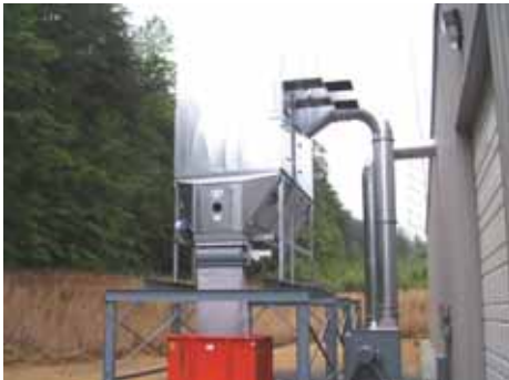
NFK On Structure / Dumping into bin
