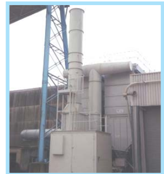
Cutting, trimming and finishing gypsum products
