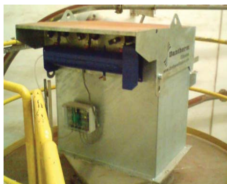
Silo venting system for dust silo, Foundry Industry
