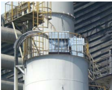
Silo venting system for dust silo, Foundry Industry
