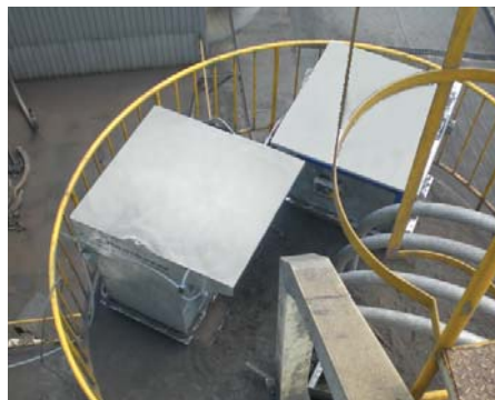
Silo venting system for dust silo, Foundry Industry
