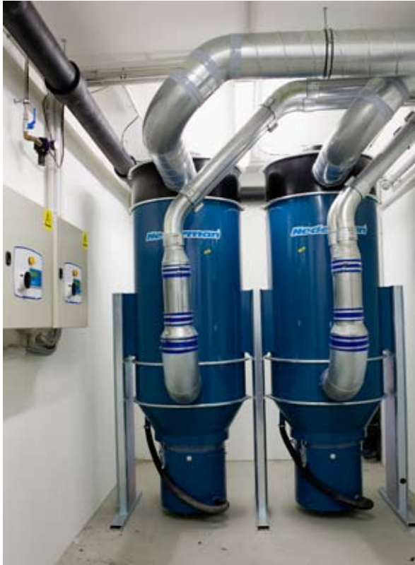
Nederman offers a full range of vacuum units for central systems including filter and duct system. The systems are designed to extract welding fumes, grinding dust, metal turnings, composite materials etc.
