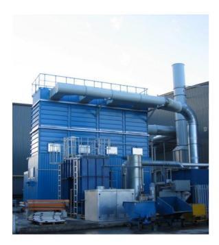
The MJB-A comprise an innovative range of robust, versatile tubular bag filter unit that build upon the experience of the well-established MJB bag filters.
