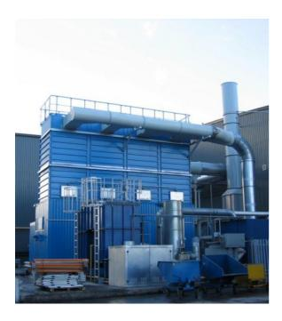
The MJB-H comprise an innovative range of robust, versatile tubular bag filter unit that build upon the experience of the well-established MJB bag filters.
