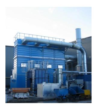
The MJB-H comprise an innovative range of robust, versatile tubular bag filter unit that build upon the experience of the well-established MJB bag filters.
