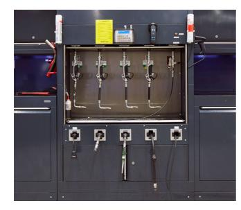
The NMS lubrication monitoring system for complete fluid control accurately monitors and supplies the correct amount of oils and liquids to each vehicle without manual handling or tapping. It also informs suppliers when it is time to refill tanks. This is the end of spillage, loss and unnecessary stoppages.
