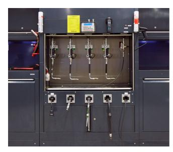
Nederman Monitoring System - NMS - is the future proof system for controlling and monitoring oil, windshield fluid and other liquids in vehicle service stations. The NMS lubrication monitoring system gives complete fluid control and accurately monitors and supplies the correct amount of oils and liquids to each vehicle without manual handling or tapping.
