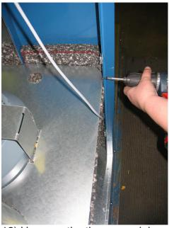
13) Unscrew the three remaining sheet metal screws securing the fan cover and remove it so it does not interfere with the fan (tilt up and out).
