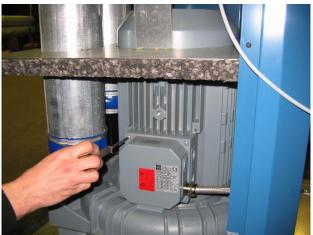
9) Disconnect the fan mains cable. (Please note and mark cables for proper re-connection). NOTE! Remove cable gland from the terminal lid. The old lid cannot be re-fitted on the new fan. NOTE! Cable shield is connected to the cable gland for proper EMC protection.
