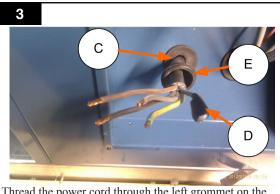
Thread the power cord through the left grommet on the cabinet as shown (C). Isolate any neutral conductor with heat shrink tape (D).
