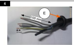
Put on the supplied rubber grommet (E). Strip the power cable insulation 10 cm. Strip the wire insulation 13mm.
