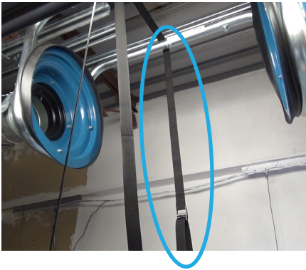
Position maintenance strap inside bolt hole pattern
