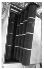
→ Pull the plastic bag with auxiliary frame over the filter module from below.
